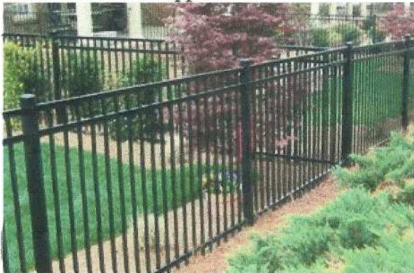
Figure 1. Typical 3 Rail Metal Fence
